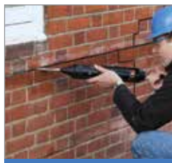
2 HeliBond-mortel in de sleuf injecteren
